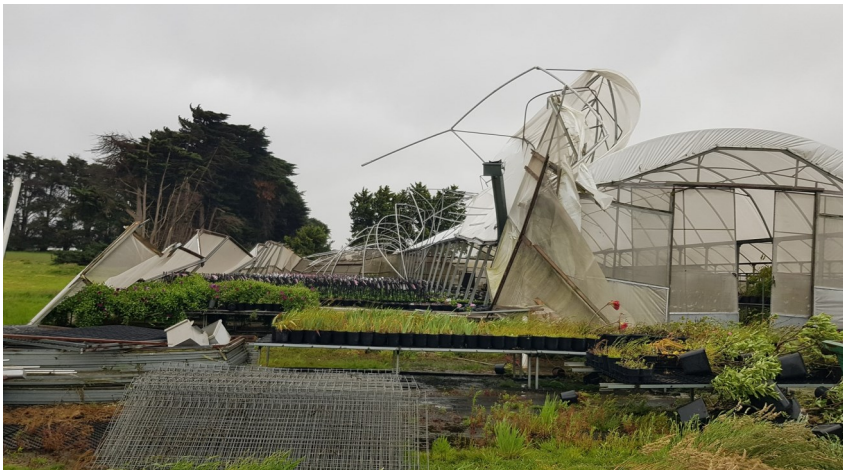
Extensive damage at Alameda Homestead Nursery
