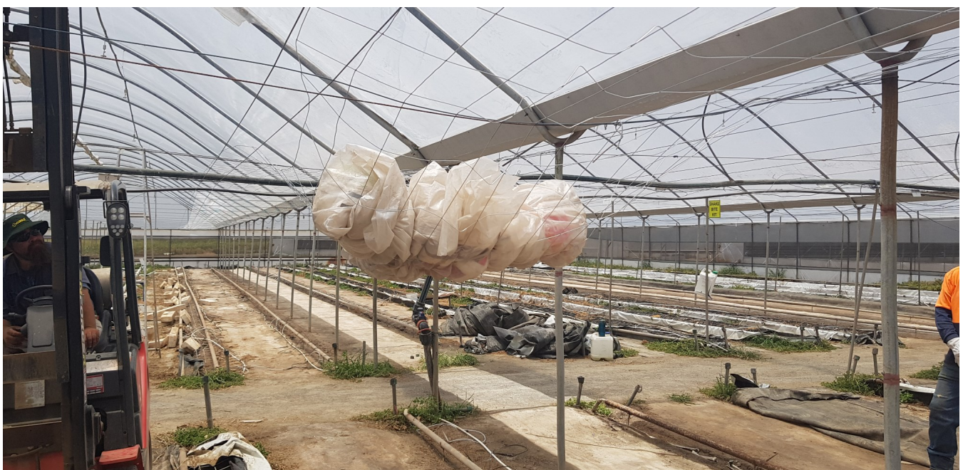
200kg of weight supported by the improvised safety net
