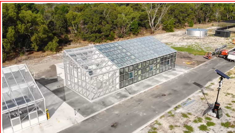
ClearVue Solar Glass Greenhouse
